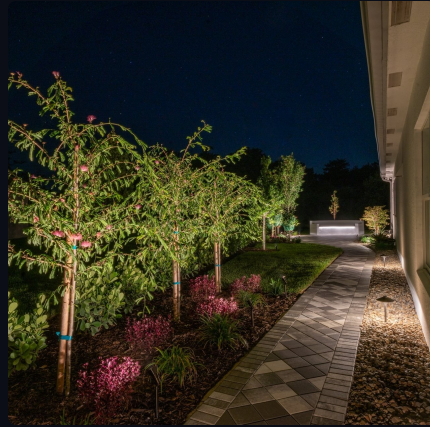
Path lights set back from the edge; the eye follows the light, not the fixture.
